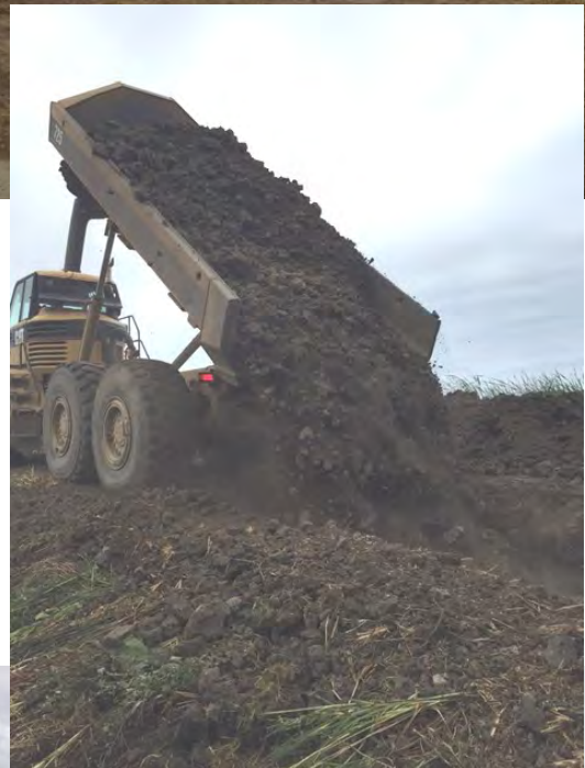
Above: Pair pond excavation to secure clay material for re-coring the dyke.
