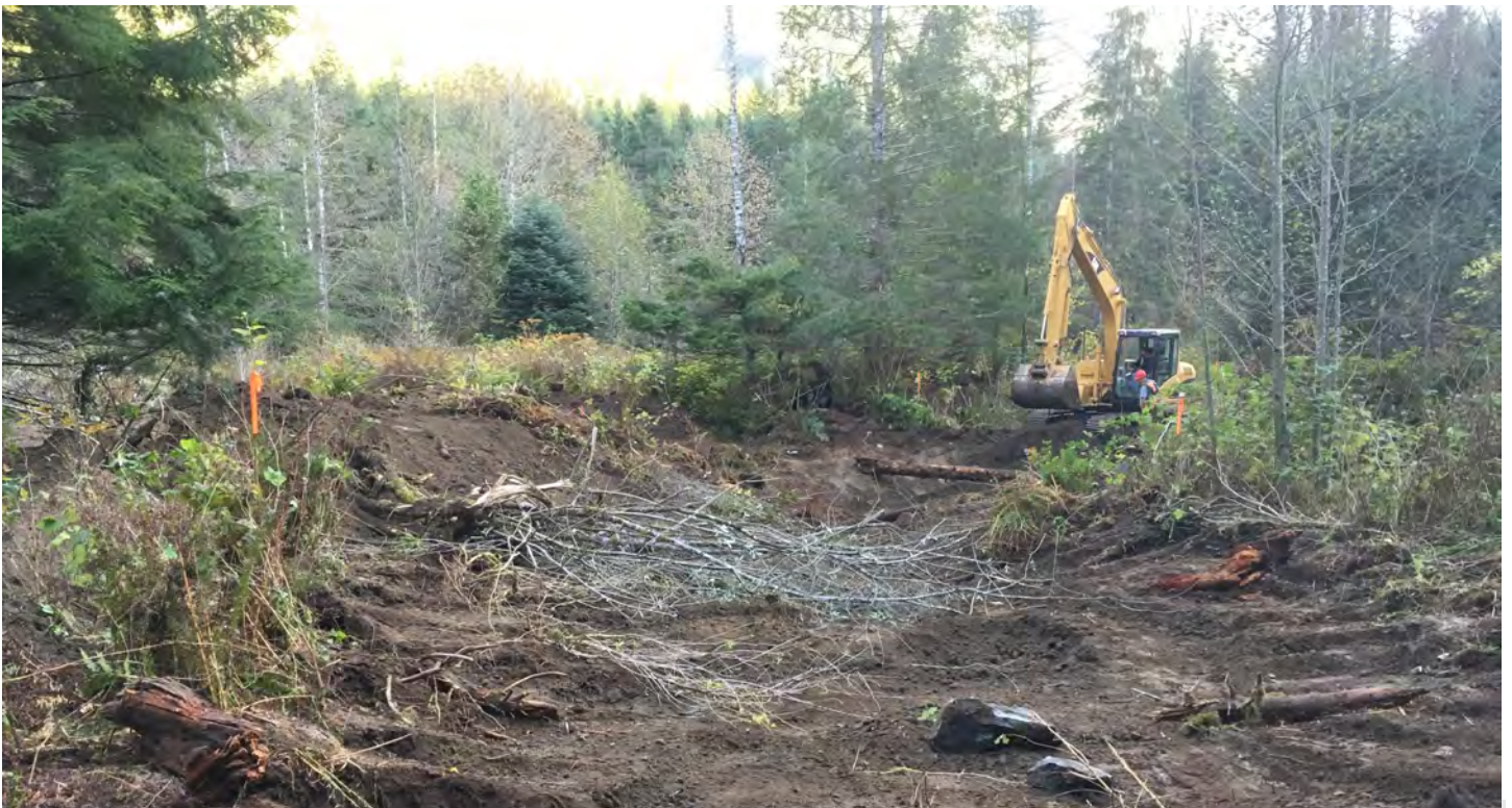
Excavating new wetland ponds in Clowhom watershed.
