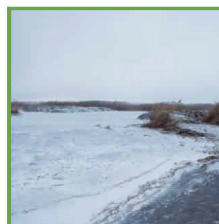
Crown Marsh east pond construction
