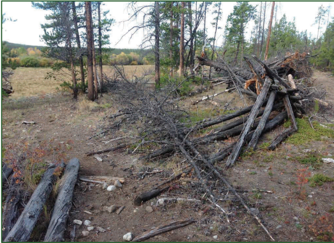
Derelict perimeter fencing to be replaced, as seen during September 2015 site visit.
