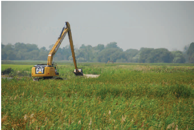
Big Creek NWA reconstruction of cross dyke (Sept. 2015)
