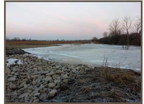
CREDIT: Lower Thames Valley Conservation Authority
