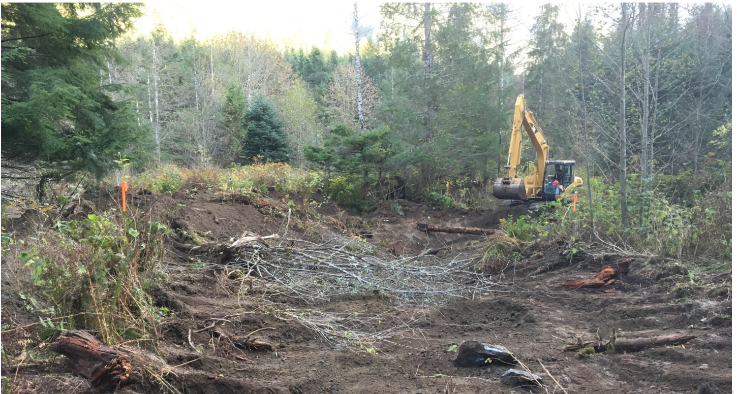
Excavating new wetland ponds in Clowhom watershed.
